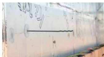
Dualfix durable spouwanker positioneren
