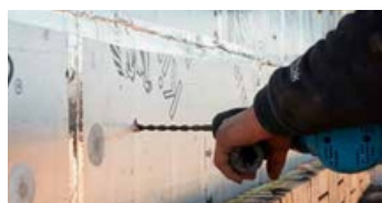
Drill 9mm: hollow materials Drill 9.5mm: solid materials
