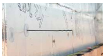
Dualfix stainless steel AISI 304 wall tie positioning
