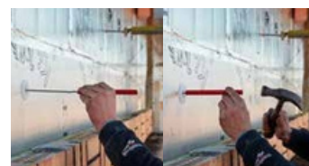
Install wall tie using suitable drift (L tie -L plug + 10 mm)
