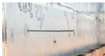
Duaflax durable spouwanker positioneren
