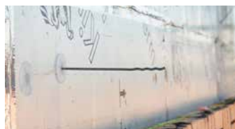
Dualfix Durable spouwanker positioneren
